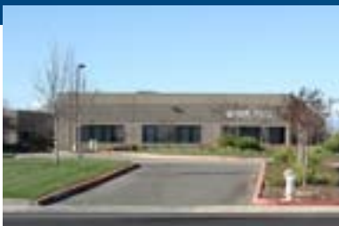
LAGUNA WEST BUSINESS PARK 3133 DWIGHT ROAD ELK GROVE, CA
